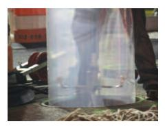
tolerance for temperatures than their steam-cured resin alternatives, but they still must be kept cool and out of the direct sunlight during the installation process. Lanzo kept the liner tubes at 60 degrees in a refrigerated trailer inside a warehouse until they were ready to use. Lanzo Trenchless Technologies completed the project on time and under budget.
