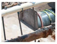
pipeline and its state of disrepair posed a significant risk of future sudden and catastrophic failure.
