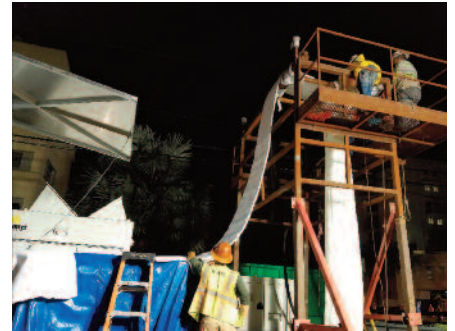
Inversion of the 20" Diameter Potable Water Lining Tube
