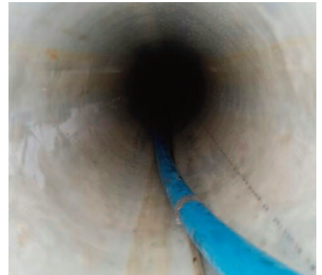
Post Inspected Defect Free and Ready for Testing
