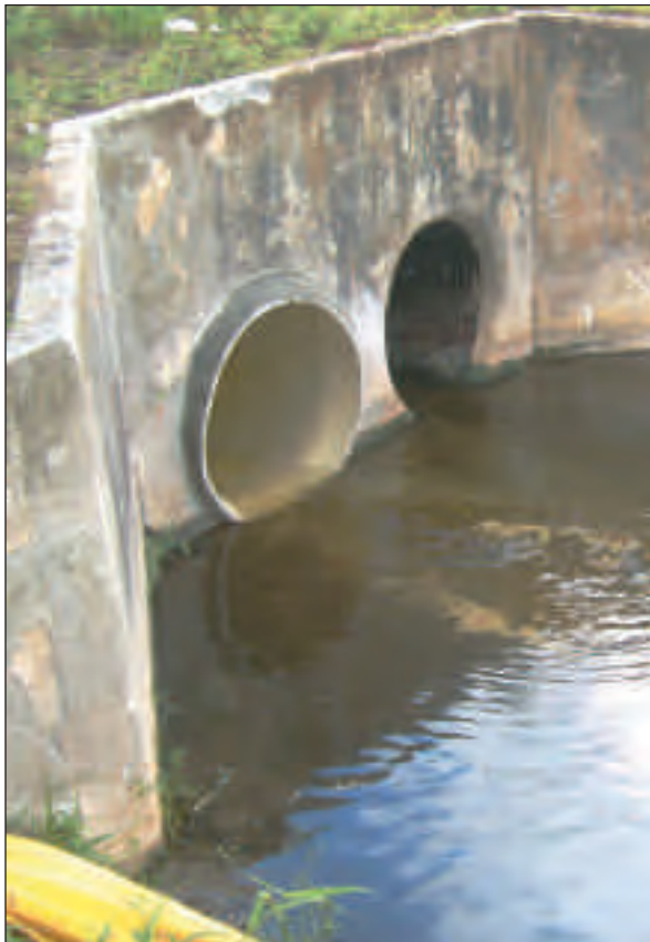
Trenchless renovation in storm drain application
