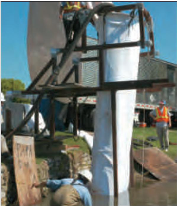
Subaqueous installation of CIPP into storm drain
