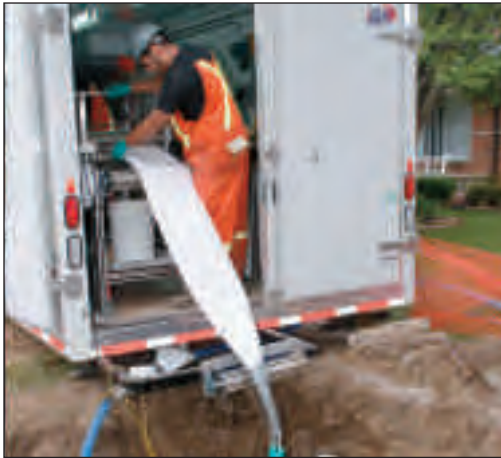
ASTM F1743 Pull & invert technology
