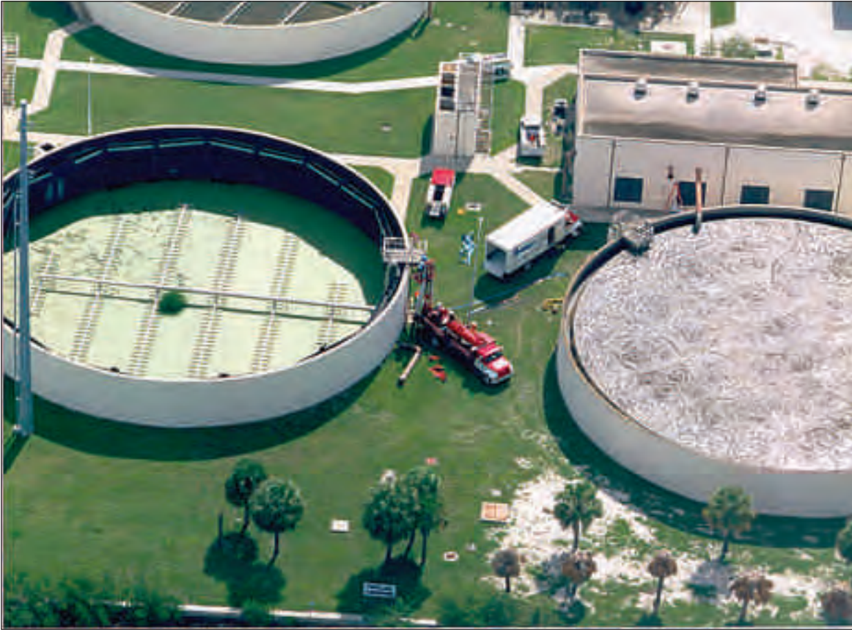
Clarifier pressure pipe rehabilitation at WWTP
