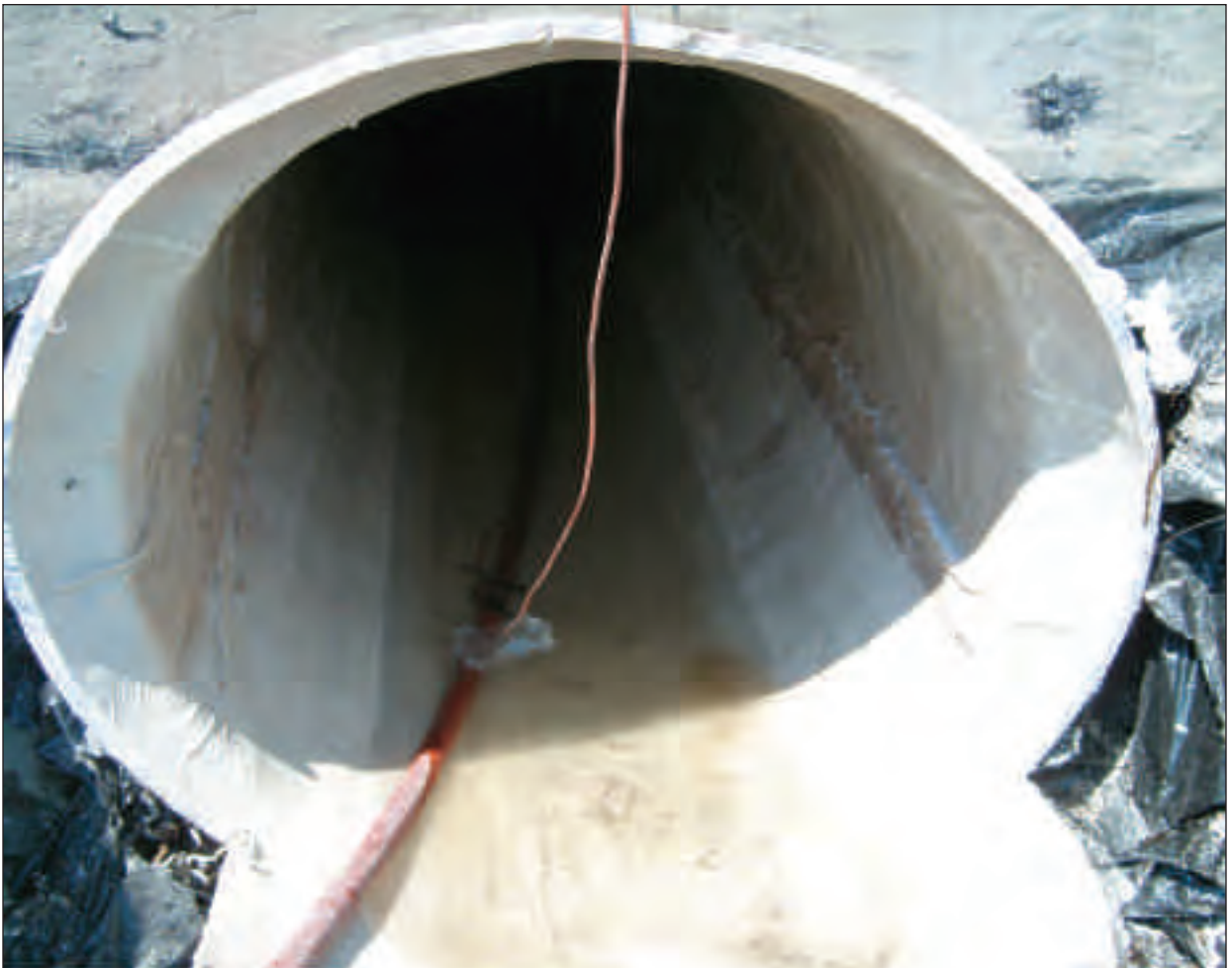
Finished outfall product at the headwall
