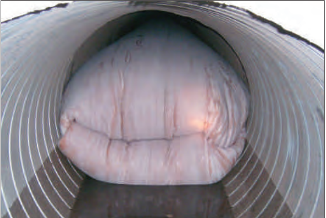
Frontal view of 60 inch diameter direct inversion
