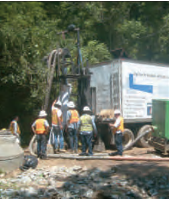
Easement installation of subdivision sewer rehab
