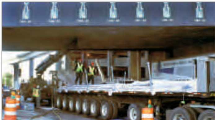
Large bore trenchless renovation in "tight quarters"
