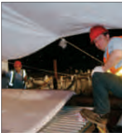
"Over the hole" wet out and installation of large bore circular, non-circular, and box culvert applications
