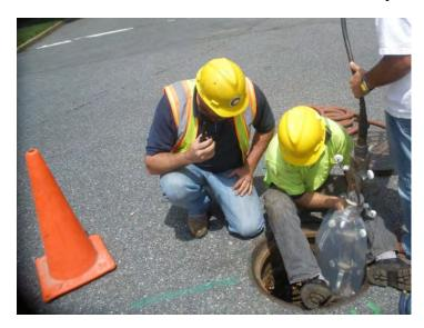
(Figure #3 Light Train inserted into a 30" Trunk Sewer on Division Street)
