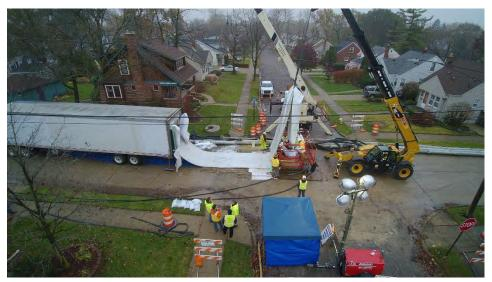
GWK was a successful installation of twin 66" diameter pipes for the Oakland County Drain Commission.
