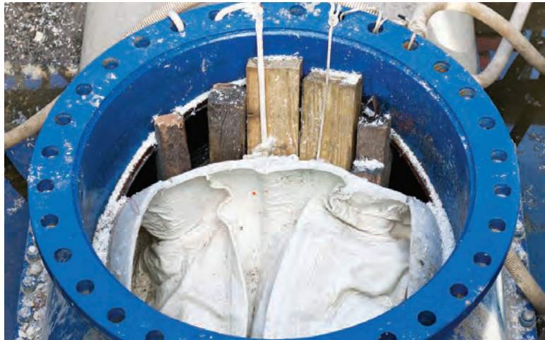
A new liner cures at the manhole opening.
